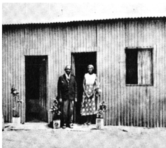
Figure 5. Malhangalene. House with walls and covering with corrugated iron foils. In: the Malhangalene Survey , 1977. p. 24.
