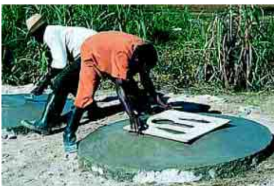
Figure 6. Concrete slabs constructions for latrines. In: National Programs of Sanitation in Mozambique: Pioneer in the Suburban Sanitation , 2002, p. 01. {www.wsp.org}.
